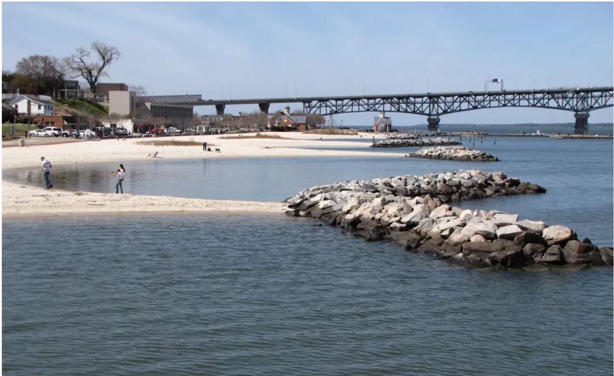
Image: A series of breakwaters promoting sediment accretion at Colonial National Historic Park, Virginia. Source: National Park Service Photo by Steve Simon, 2012
