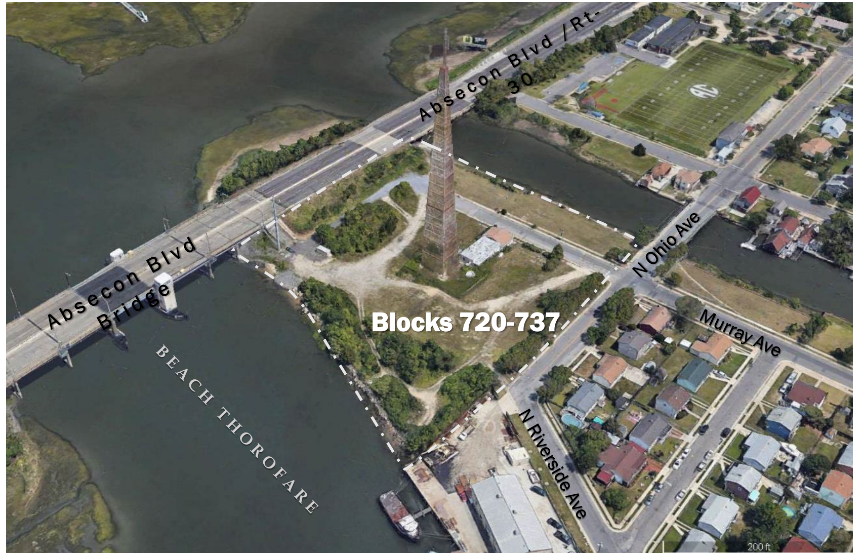
Aerial view of 1817 Murray Avenue from the west (source: Google Earth)
