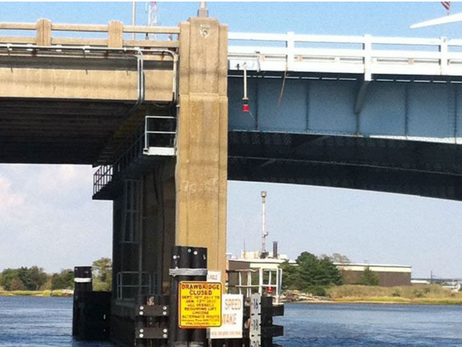
Absecon Boulevard Bridge, during its 2012 renovation. Source: IEW Construction Group, www.iewconstructiongroup.com/
