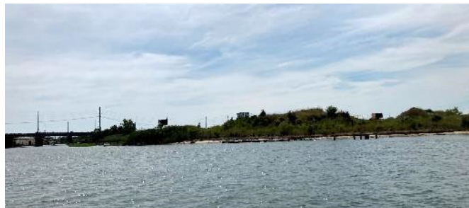
2141 Absecon Boulevard from the water (Photo by Perkins Eastman)
