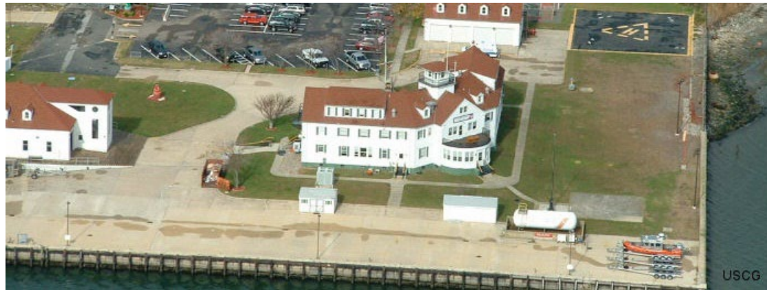
Existing Buildings, Coast Guard Air Station (CGAS) Site
