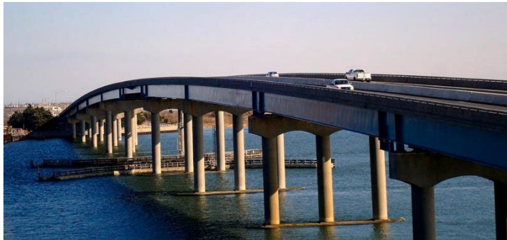
Brigantine Bridge (photo by Arlane Crump, 2017)
