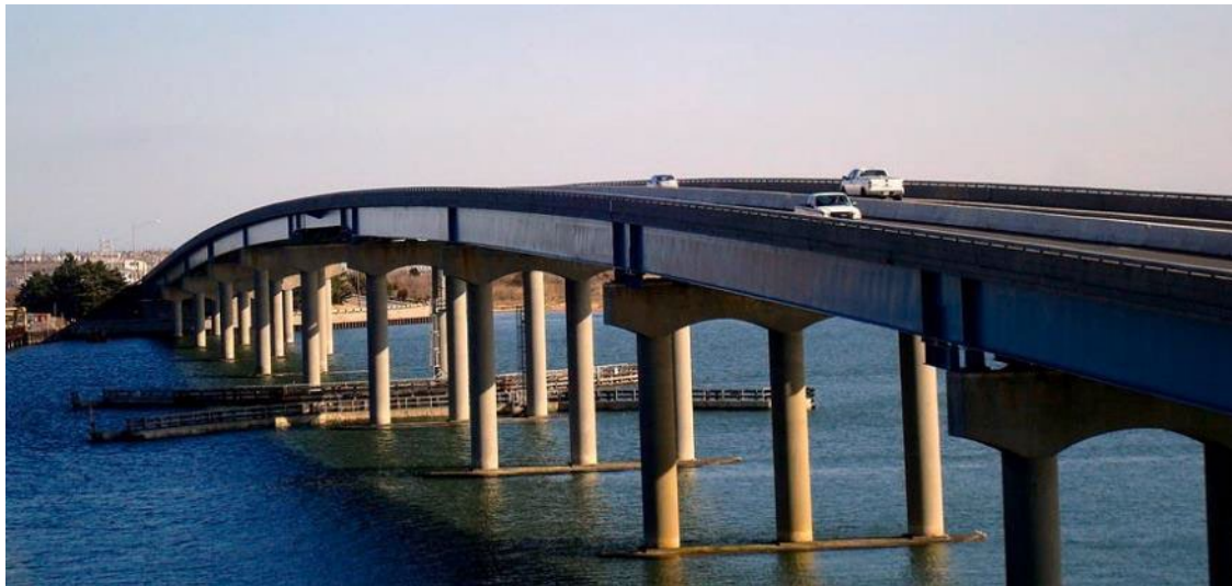
Brigantine Bridge (photo by Arlane Crump, 2017)
