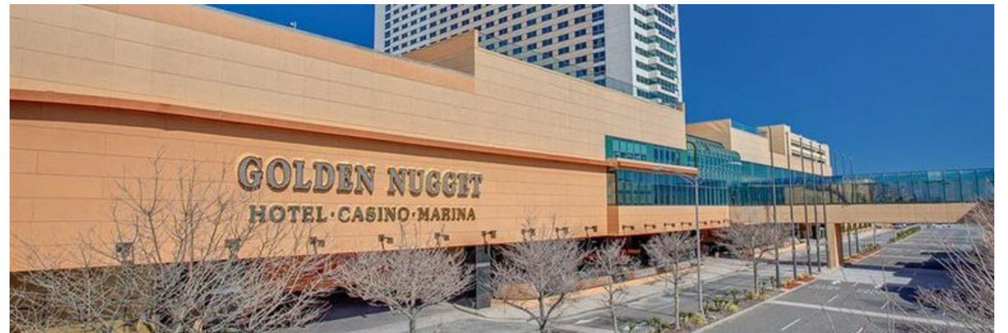
Huron Avenue looking north (source: www.travelagewest.com)
